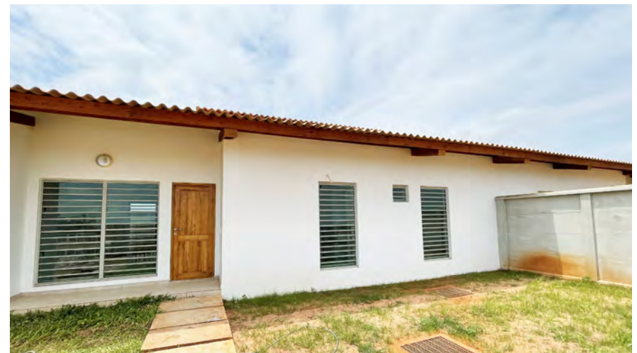
Figure 1 Cité Ouèdo, 20,000 Logements under construction, Center Lane, July 2023 (Olufèmi Hinson Yovo)
